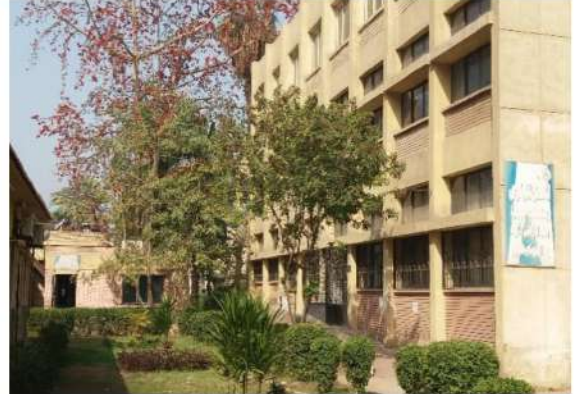
Three-floor Central Lab Building
