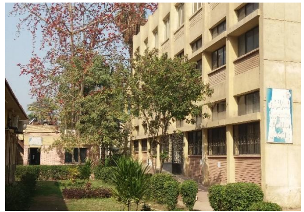
Three-floor Central Lab Building
